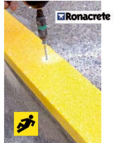
Mechanical fixing of the nosings
