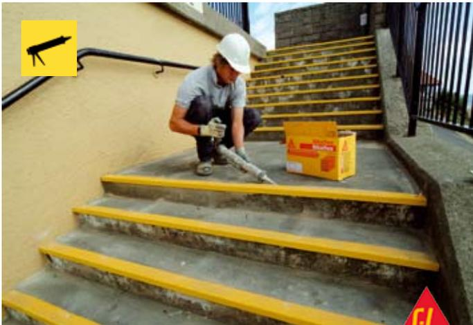
Final sealing with Sikaflex 11FC adhesive sealant to the nosings
